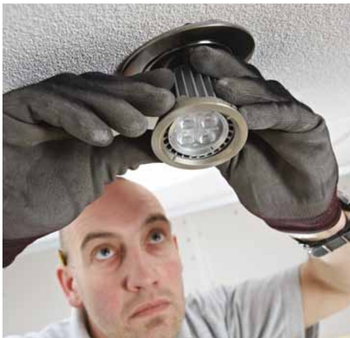
Julian Evans, Fullcircle Electrician installing Carbon Trust Approved LED
