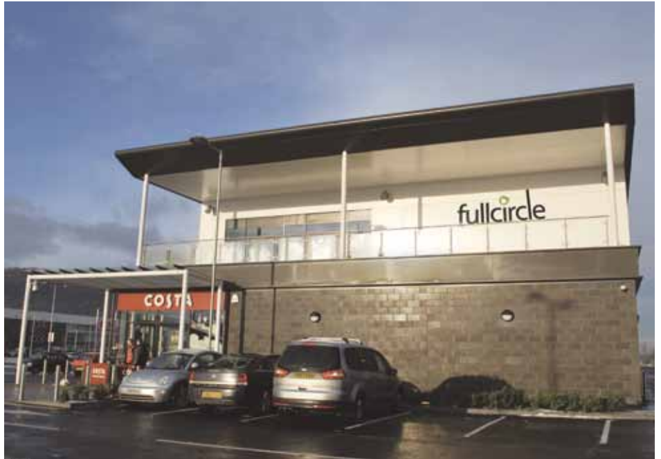
The Pod, Capital Retail Park - Fullcircle Head Office
